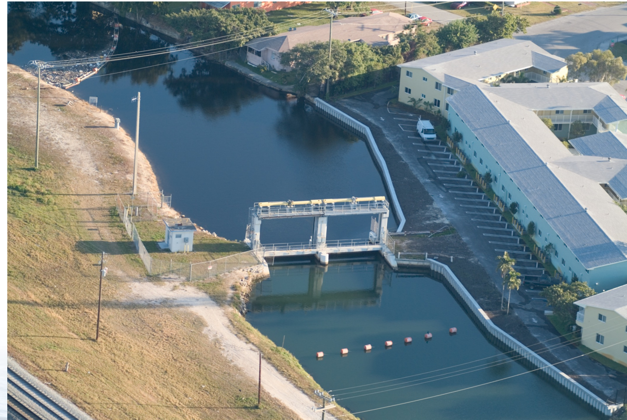
S-27 Structure – Gated Spillway
