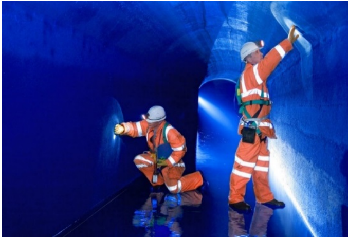
Maintenance of an aqueduct (Credit: United Utilities)
