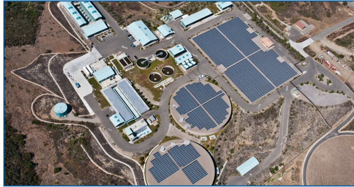
Solar Panels at the Twin Oaks Valley Water Treatment Plant
