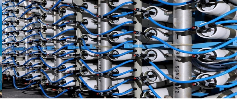
Carlsbad Desalination Facility (left) and reverse osmosis membranes at Carlsbad Desalination Facility (right)
