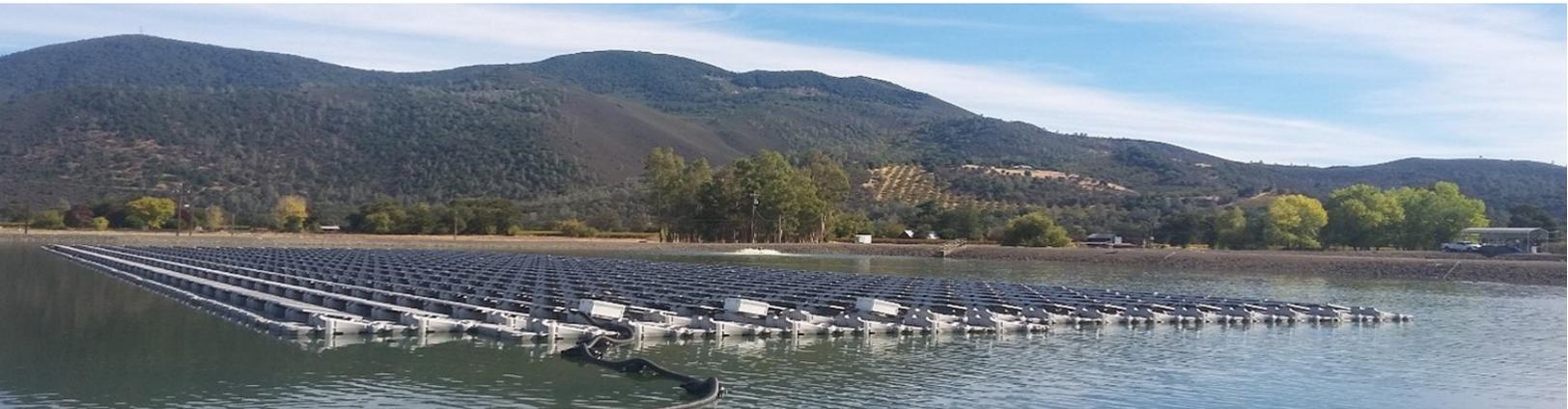
*The floating solar array installed on a polishing pond for one of Lake County Special District's treatment plants*
