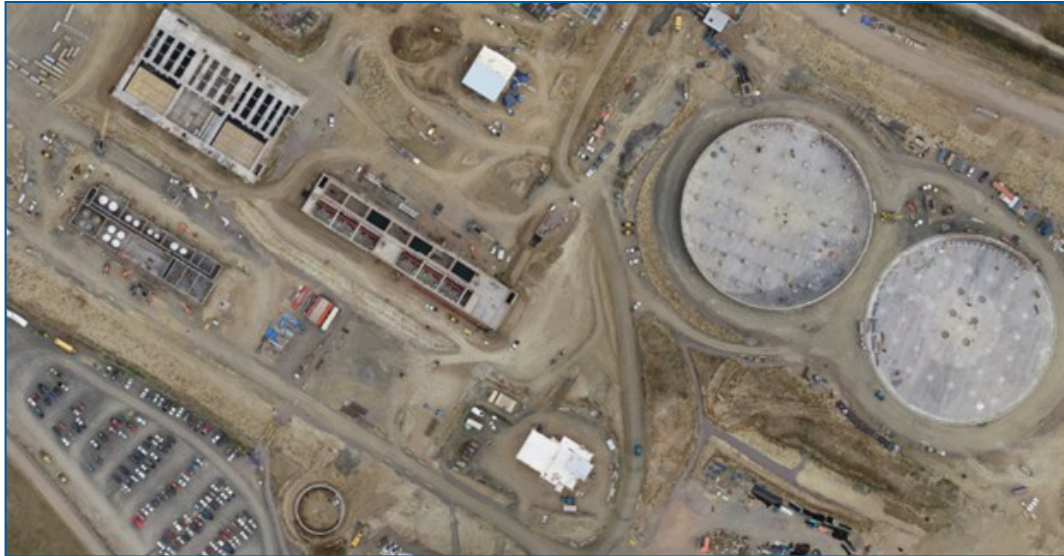
Aerial View of Denver Water's sustainable Northwater Treatment Plant under construction
