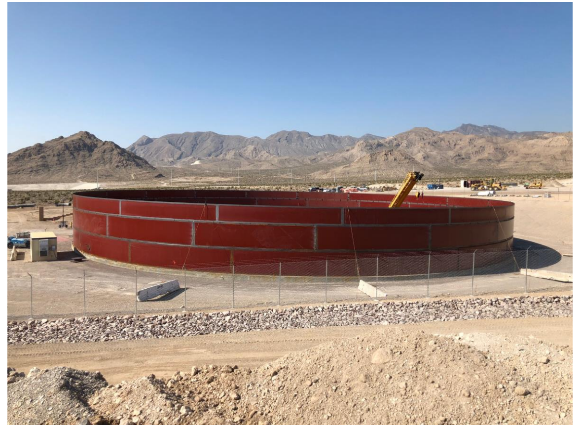
Interim above ground steel storage tank Las Vegas, NV
