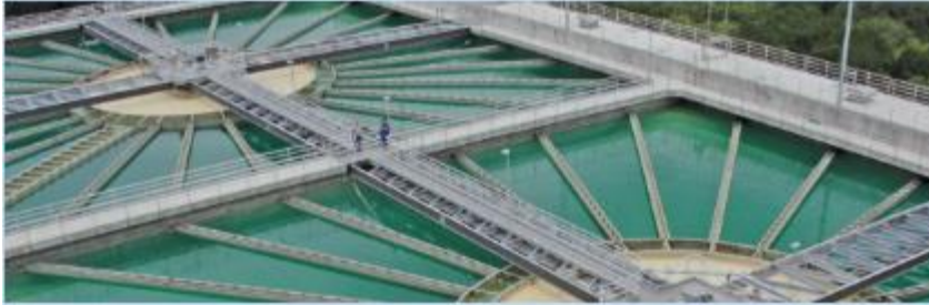
Davis Water Treatment Plant
