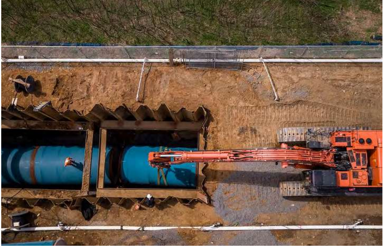
Planning informs PWD's investment in large-scale infrastructure
