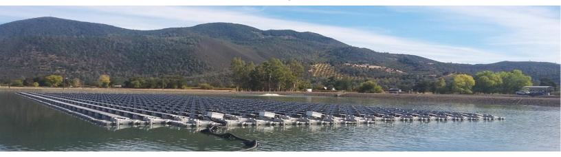
The floating solar array installed on a polishing pond for one of Lake County Special District's treatment plants
