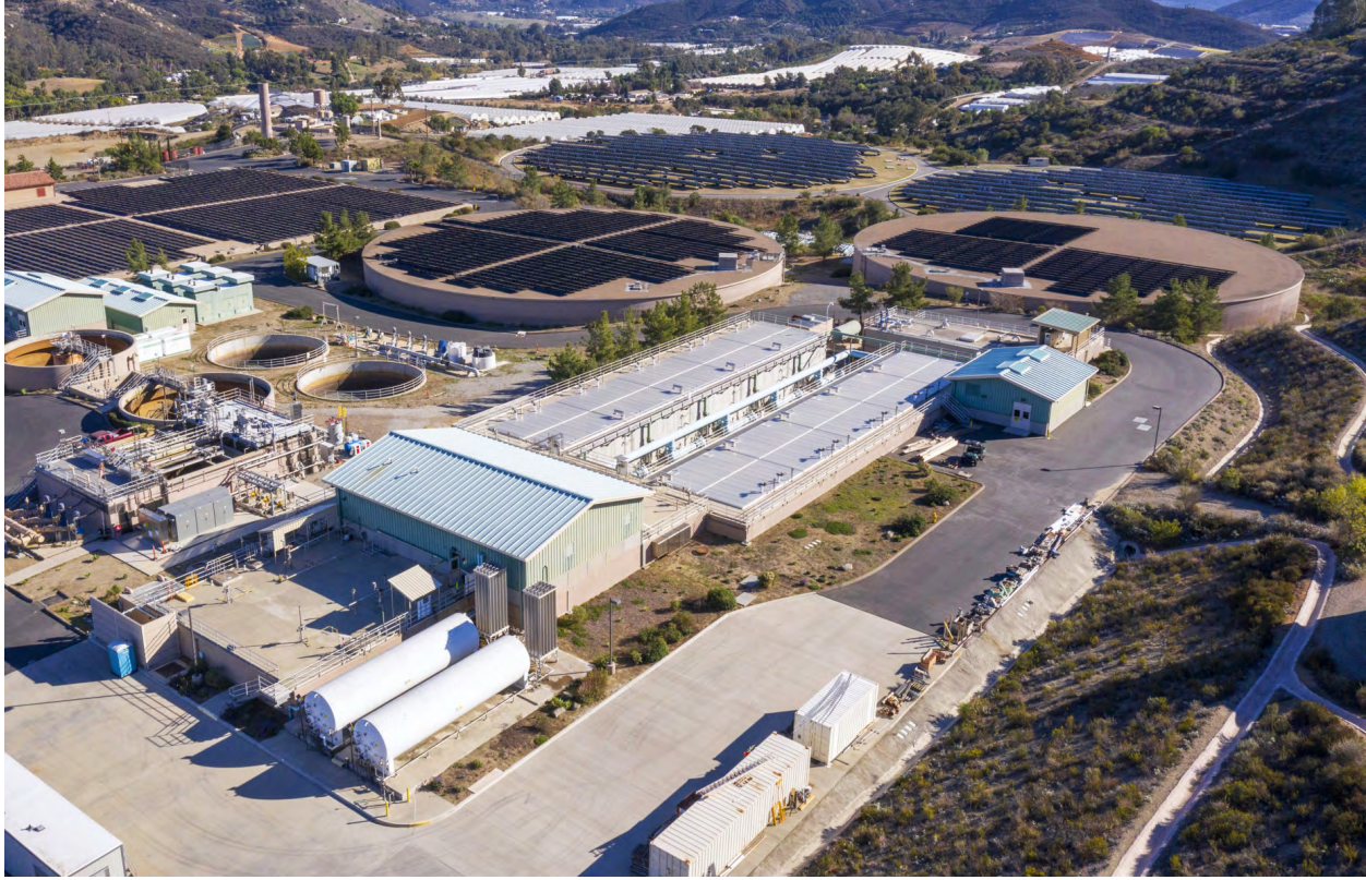
Twin Oaks Valley Water Treatment Plant
