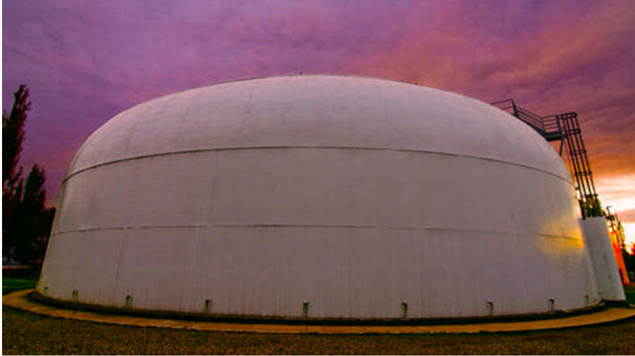
Infrastructure in Portland's groundwater well field
