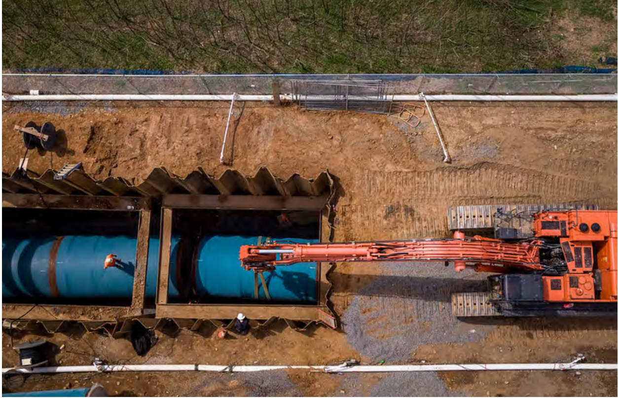
Planning informs PWD's investment in large-scale infrastructure
