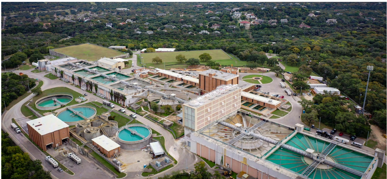
Ullrich Water Treatment Plant, the largest of Austin Water's three water treatment plants
