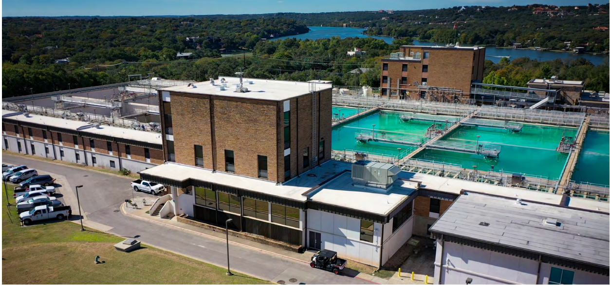
Davis Water Treatment Plant, with Lake Austin in the background
