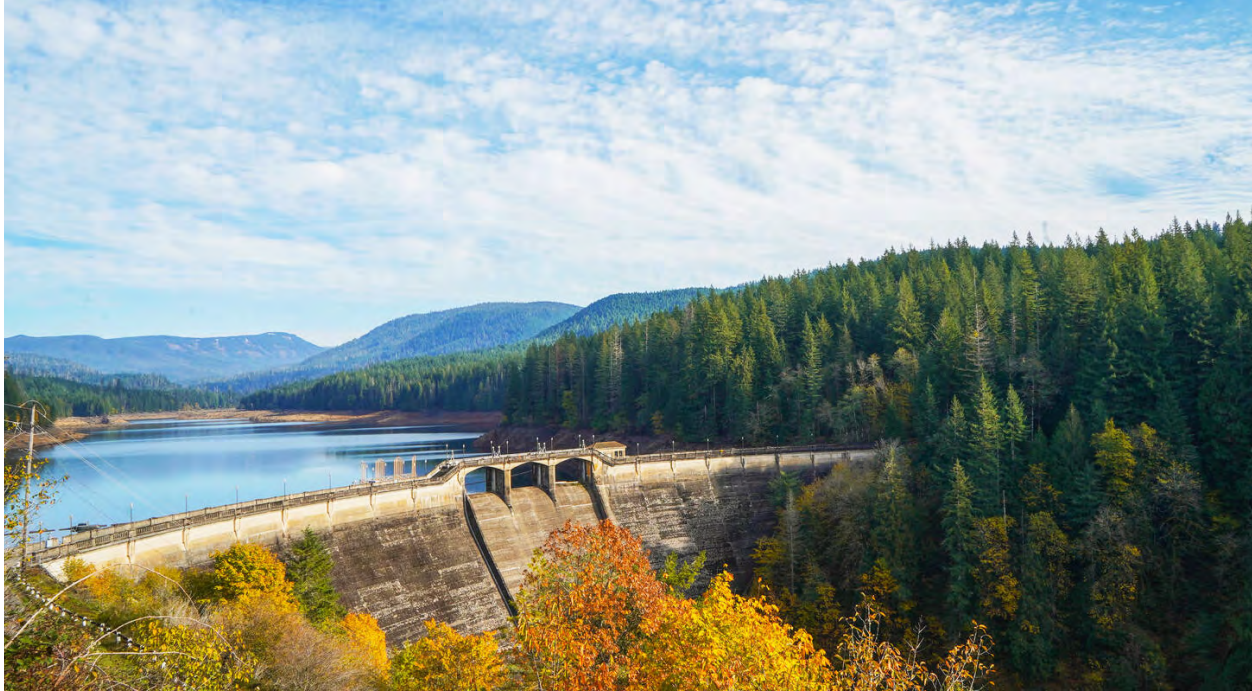
Dam 1 and Reservoir 1, Bull Run Watershed
