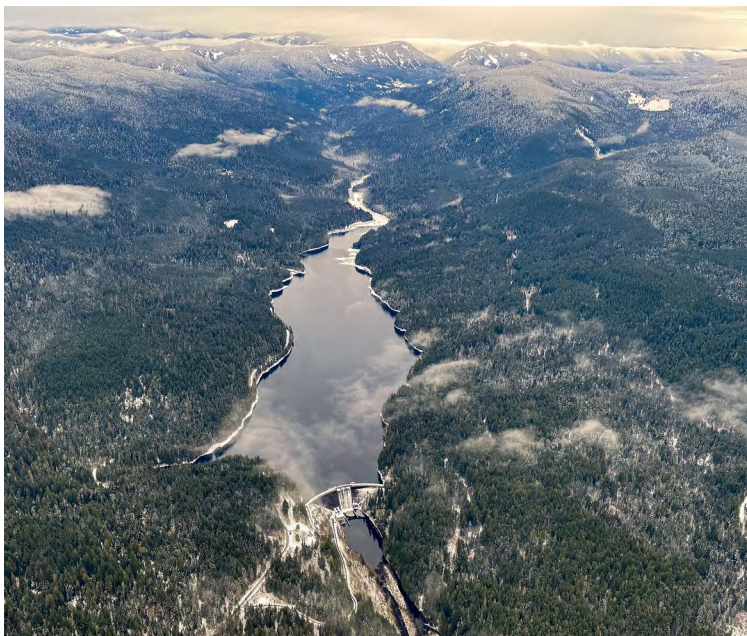
Aerial view of Bull Run Reservoir #1 and the upper Bull Run Watershed, February 2025. (Image: Wikipedia user Tedder, under CC BY 4.0 .)
