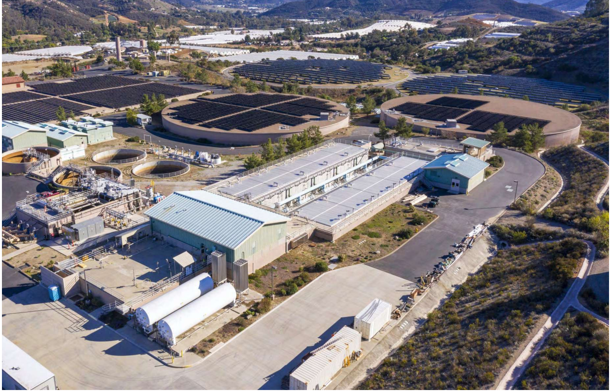
Twin Oaks Valley Water Treatment Plant
