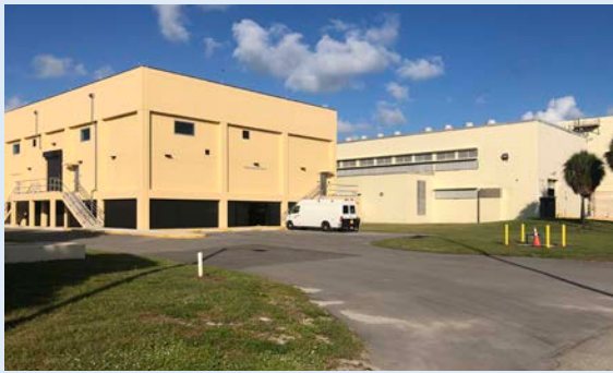
Central District Wastewater Treatment Plant Facilities Image Courtesy of Miami-Dade County
