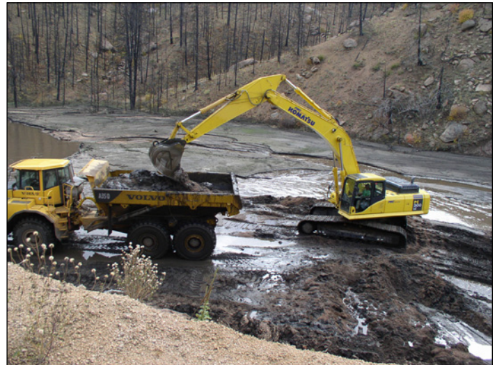
Sediment is removed from Turkey Creek in the Upper South Platte Watershed. (Courtesy of Colorado State Forest Service)
